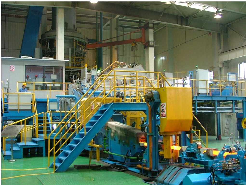
View from the CONTIROD ®* line to the shaft furnace.
