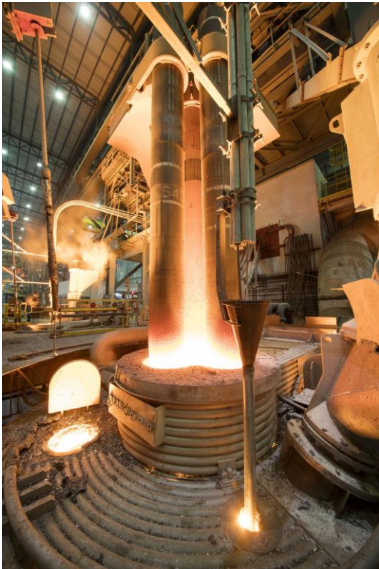
Twin-ladle furnace (LF) in operation.
