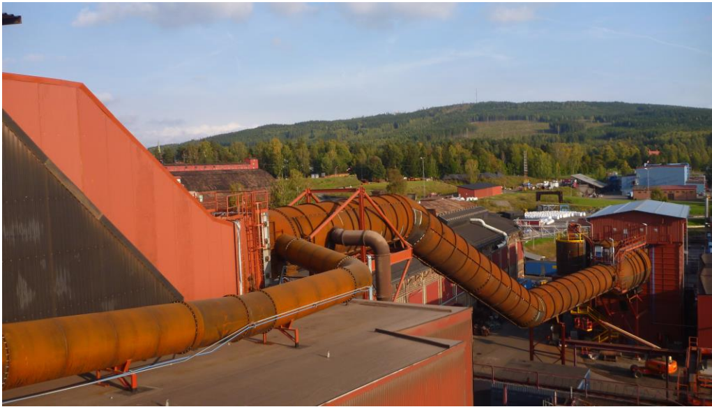
New secondary and inlet duct to the filter unit supplied by SMS group.
