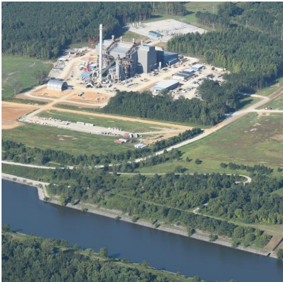
The works of Mississippi Silicon, USA, with two submerged arc furnaces and Ecoplants environmental technology from SMS group.
