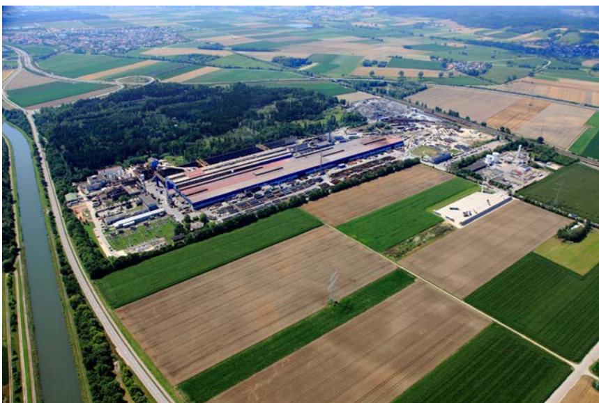
Lech-Stahlwerke in Meitingen, Germany (Source: Peter Viskomm).
