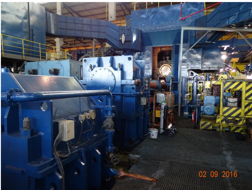
Drive side of the rolling stand after the repair.
