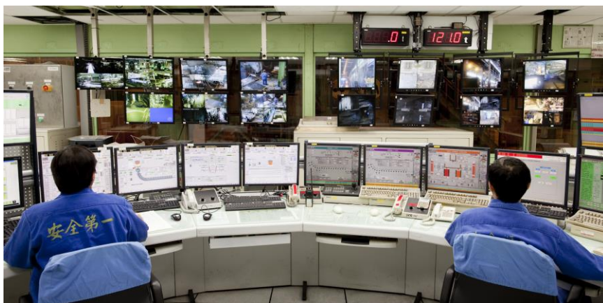
Main control pulpit on the casting deck of the two-strand continuous slab caster No. 7, China Steel Corp.
