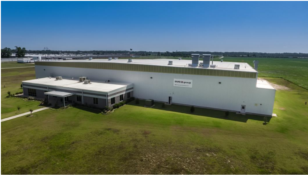
New workshop operated by SMS Technical Services in Osceola, in the southern U.S. state of Arkansas.
