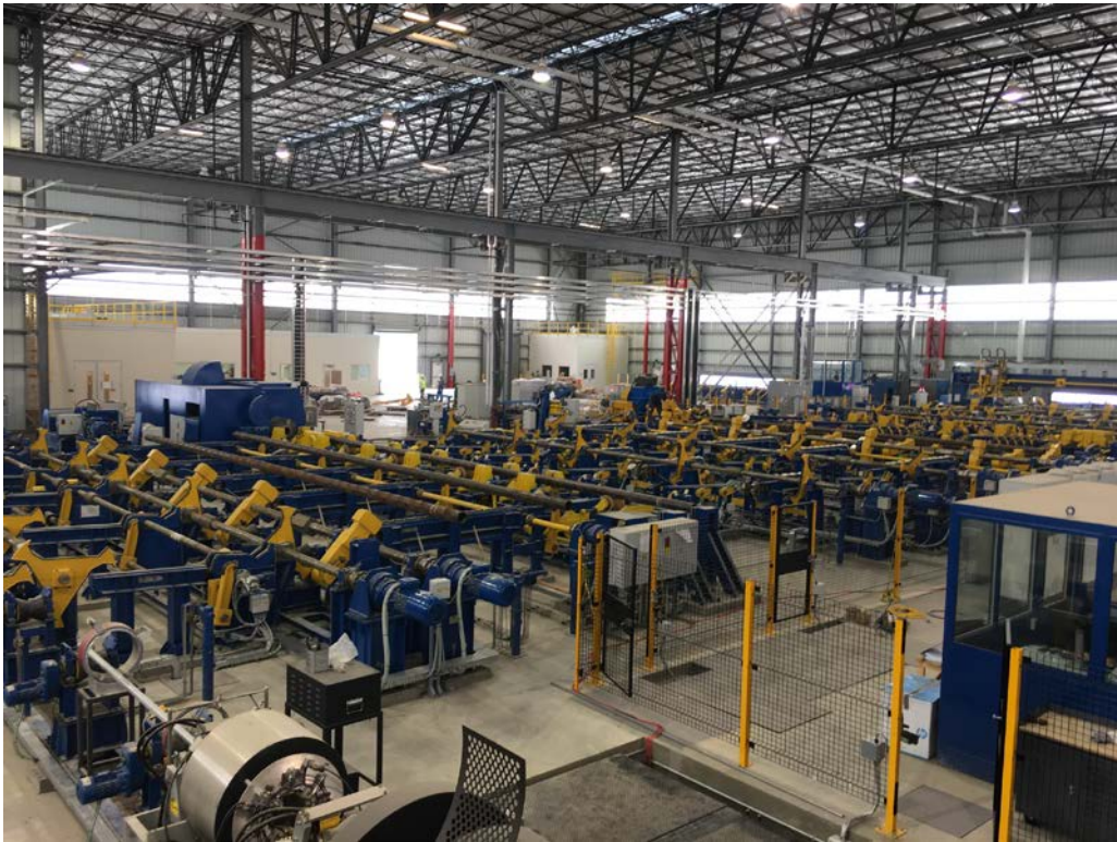
CNC threading machines supplied by SMS group in operation at Axis Pipe and Tube.
