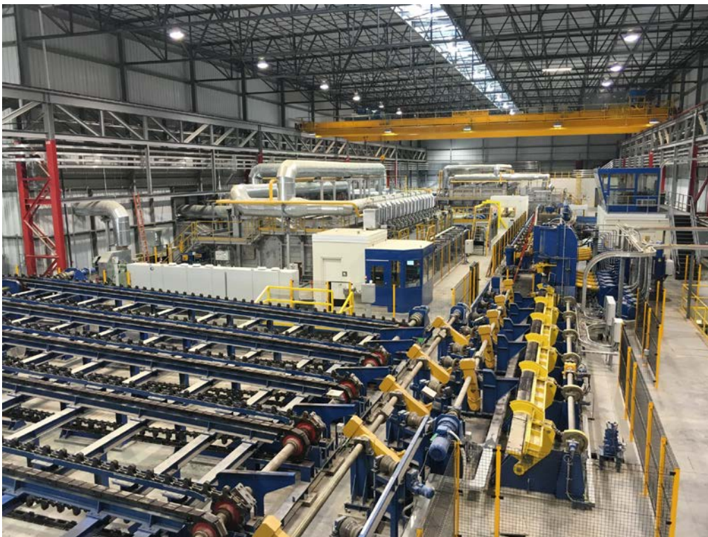
SMS group heat treatment line in operation at Axis Pipe and Tube.
