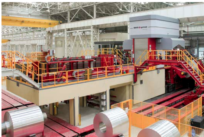
Aluminum cold rolling mill built by SMS group.
