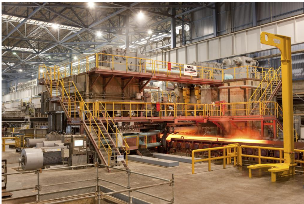
Similar slab sizing press for slab width reduction in one pass.
