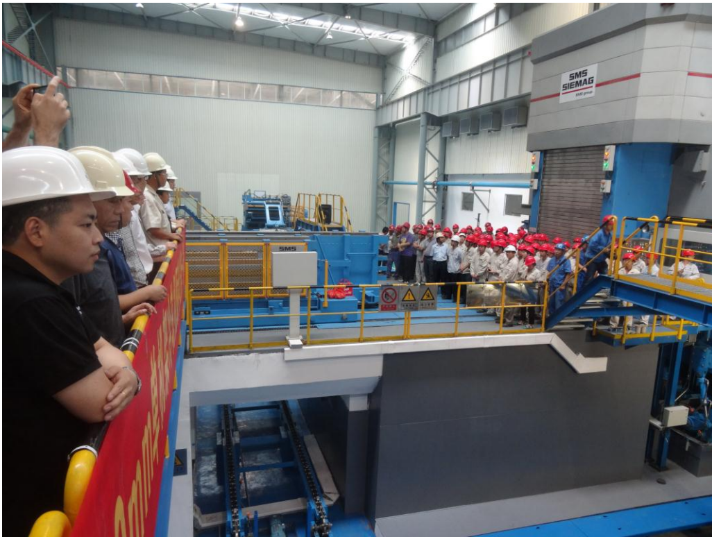
An exciting and festive moment for everybody involved: the start of operations on the single-stand cold mill at Henan Yulian.
