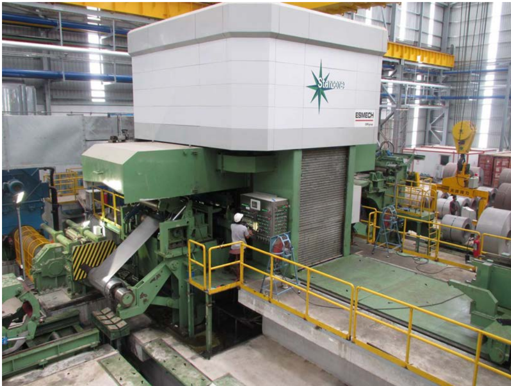
The new combined rolling and skin-pass mill at Starcore.
